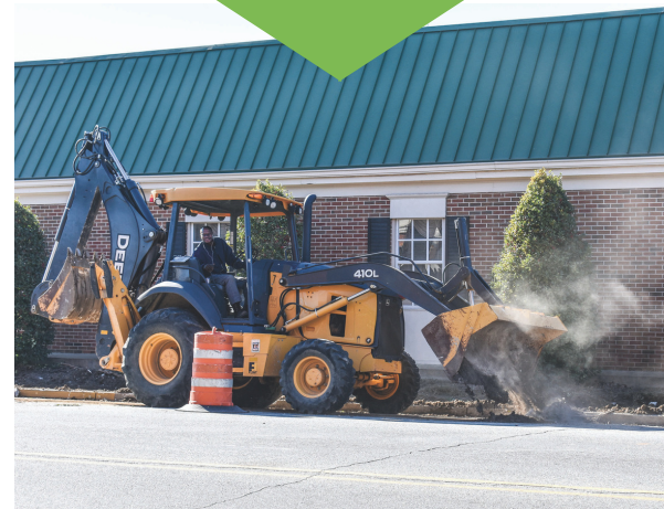
New Sidewalk Construction Underway Photo credits to Angela Barentine, The News Observer Managing Editor
